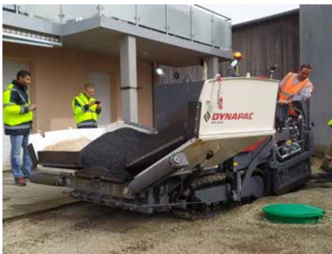
Paving in tight/narrow situations
