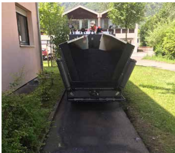
Paving bicycle path, trenches and side walks
